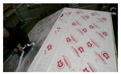
Here you can see a roof fully fitted with the insulation board and the joints all taped up with the foil tape. Then next the OSB board needs fitting over the top of the insulation board.
