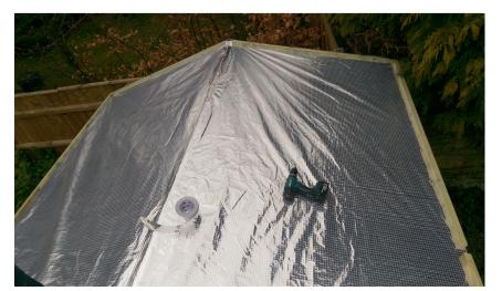
You can see the perimeter edge batten fixed on this log cabin at the bottom of the roof and the gable ends to the ridge. They can be fitted on top of the membrane too to help hold it flat on the roof. This will stop it lifting in the wind, whilst you complete the insulation kit installation
