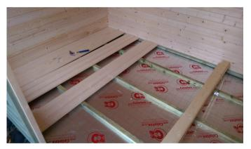
Once the insulation has begun between the floor joists, you should begin laying your cabin floor boards. If you lay part of the insulation in the floor and then board over it with your cabin floor boards you won't need to worry about standing on the insulation board and accidentally pushing down past the screws and damaging it. Do the insulating and the laying of the floor boards simultaneously, for the best results.
