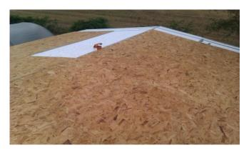
Here you can see the roof almost completed and ready for the felt or felt shingle tiles to be fitted.
