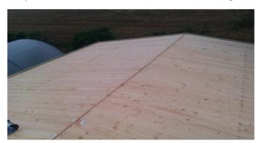
This image shows the log cabin roof boarded with the t&g roof boards, supplied with a typical log cabin. These are usually 18mm-20mm thick in good quality buildings.
