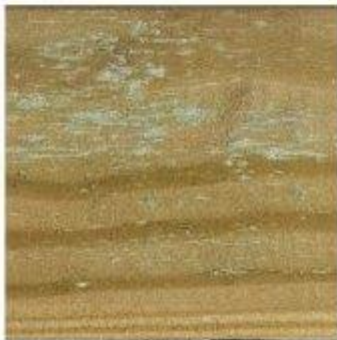
Pressure treated timber with some speckling left by the treatment salts.
